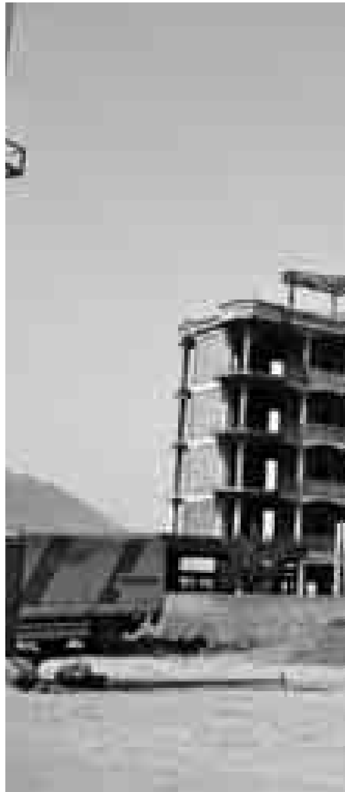
Building site in Shkodra, between Tirana and Podgorica, Azra Aksamija
